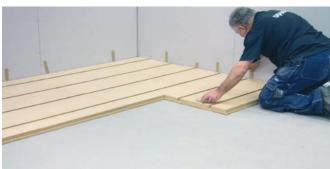
The Uponor Calma components ensure a smooth and easy installation process that is fully compliant with all relevant construction norms and regulations. The pipes are positioned and fixed in place in the heat emission plates. These features not only ensure that heat output is transferred exactly as calculated, they also enable precision temperature control and lead to substantial savings on energy and operational costs.
