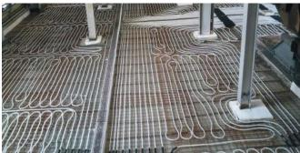
Uponor Magna industrial floor heating and cooling is integrated directly in the concrete floor slab. In the process the existing mat reinforcements can be used to fasten the pipes. Both conventional hot water heating systems and regenerative heat generators and equipment for waste heat utilisation from industry processes can be used to heat the heating water.
