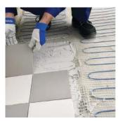
Laying Uponor's Comfort E system couldn't be easier – the mats are simply rolled out on the prepared substrate. The self-adhesive underside of each cable mat ensures that they securely bond to the substrate. Tiles can then be laid with tile cement directly on top of the heating system. Once the tiling has dried and been grouted, the Uponor Comfort E system is ready to use, generating cosily comfortable underfloor heating.
