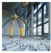
Uponor Classic wet construction system is the ideal underfloor heating and cooling system for variable flooring structures in new residential building construction and in the commercial field. Three different mat grids make optimal adjustment of the heating pipe spacing to the respective heat requirements possible. In combination with high-load insulation materials the Uponor Classic wet construction system can also be used in areas subject to high service loads.
