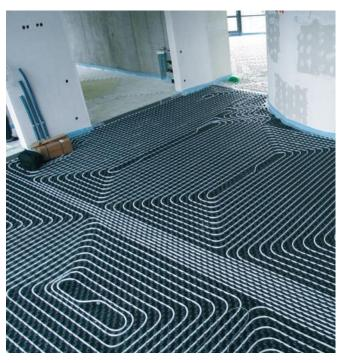
Uponor Tecto nub panels are used for the installation of underfloor heating/cooling systems in residential buildings and in commercial areas. They are installed in the floor structure below a load distribution layer made of cement or anhydrite screed. These are available in two different versions (ND 30-2 and ND 11) for different floor structures and loads.
