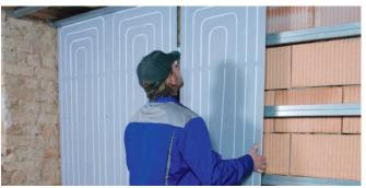
The Uponor Renovis radiant heating/cooling system consists of a gypsum plasterboard in which the Uponor PE-Xa pipes have already been integrated in the factory. It allows the temperature control of rooms via walls and ceilings in dry mortarless construction. An extensive Uponor range of products is available for professional interconnection of the panels in accordance with the Tichelmann principle.
