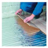
In dry construction, first the Uponor Comfort E aluminiumfoil heating mats are rolled out. Optional insulation panels prevent any damaging of the mat underside while also reducing downward heat loss. Once the Comfort E heating system has been laid, the suitable floor covering can be laid atop it immediately.
