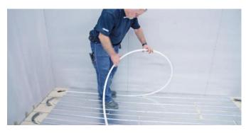
Uponor Tignum is used for quick installation on joist directly in a timber floor approx. 600 mm. It is flexible to use since it is suitable for many "on joist" floor constructions.
